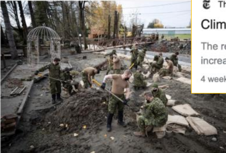
Members of the Canadian Forces fill sandbags to create a makeshift dike behind houses in Abbotsford, British Columbia, where last month's rainfall led to catastrophic floods. PHOTOGRAPH BY DARRYL DYCK, THE CANADIAN PRESS/AP
